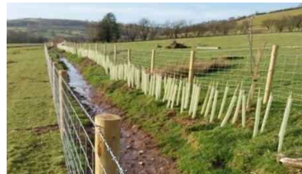
New hedge with ditch reprofiled as a swale which will slow the flow over time
